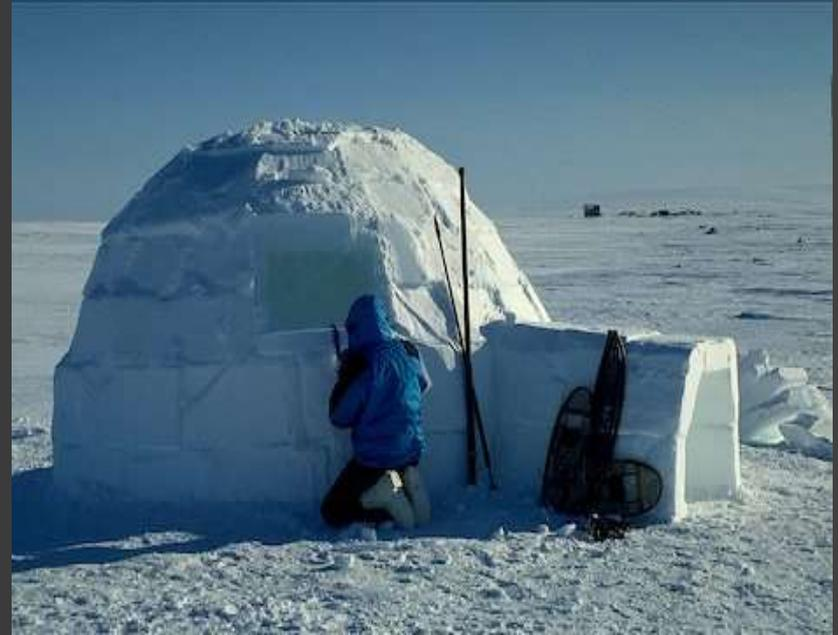
Made of ice bricks with thickness of about 500mm. The indoor temperatures can be maintained at above  $-5^{\circ}\text{C}$  when the outside temperature is  $-30^{\circ}\text{C}$ .
