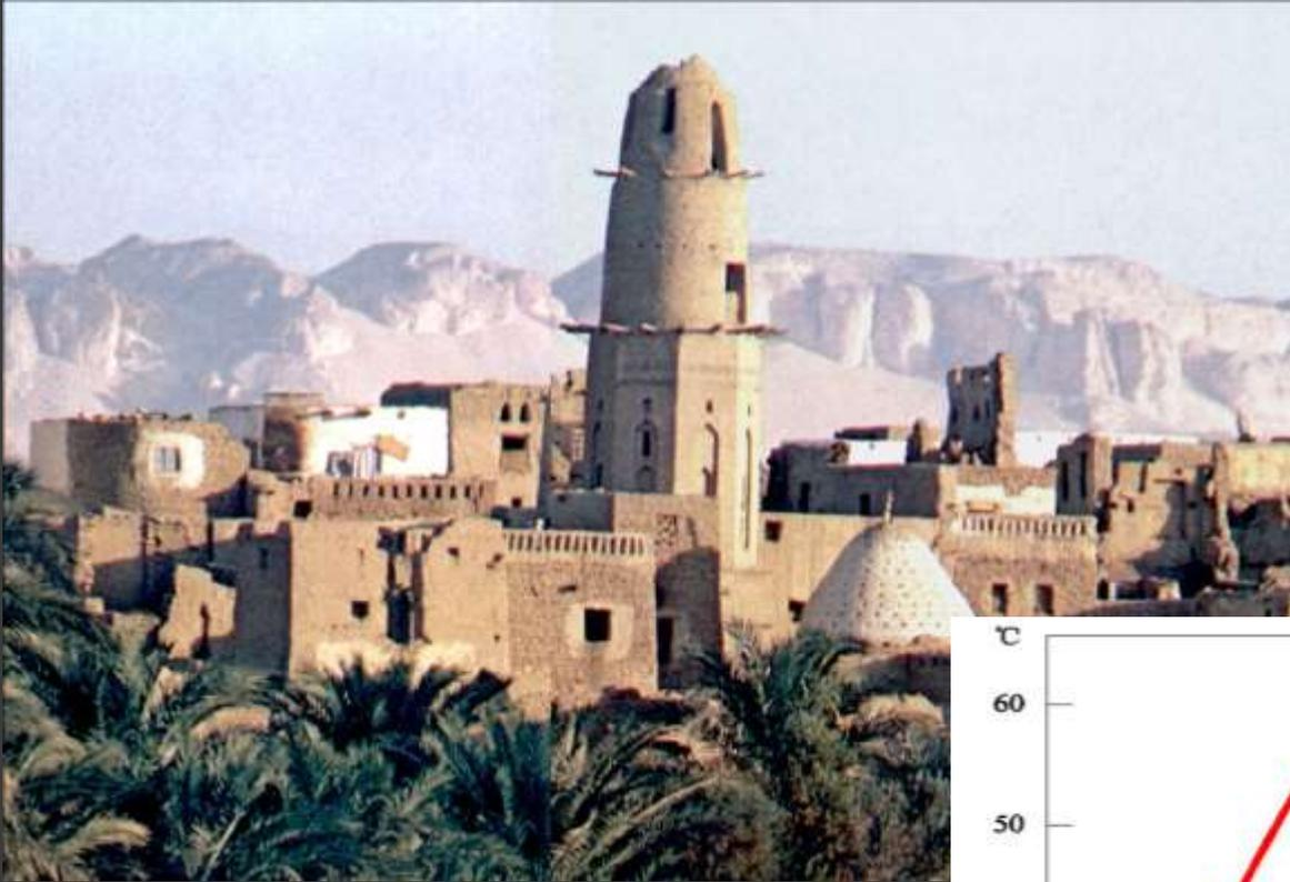
Brick thickness is more than 400mm. Due to the big thermal mass, indoor temperature difference in a day is less than 6°C, while outdoor temperature difference is more than 24°C.
