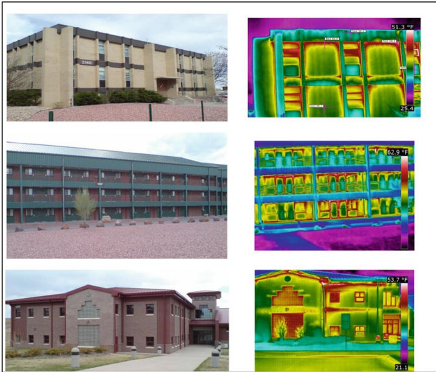
**Fig. A.2** Examples of thermal bridges: parapets, doors, slabs
