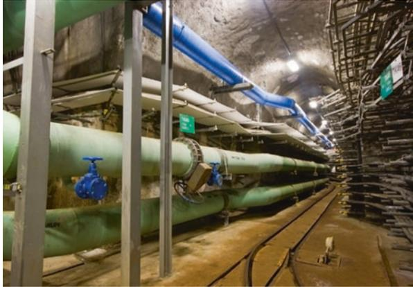
Fig. F.62 District heating development and concrete duct (utility tunnel)
