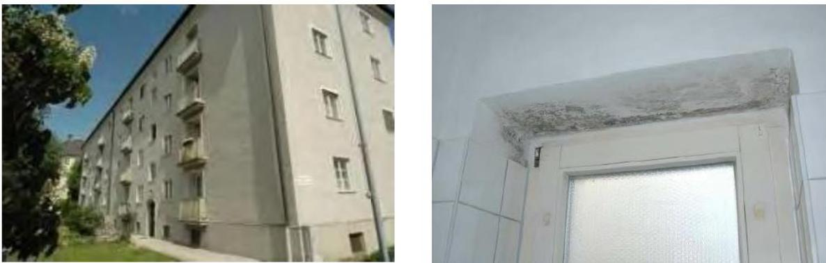
*Figure 2. Photographs of the conservation state of the buildings prior to rehabilitation*
