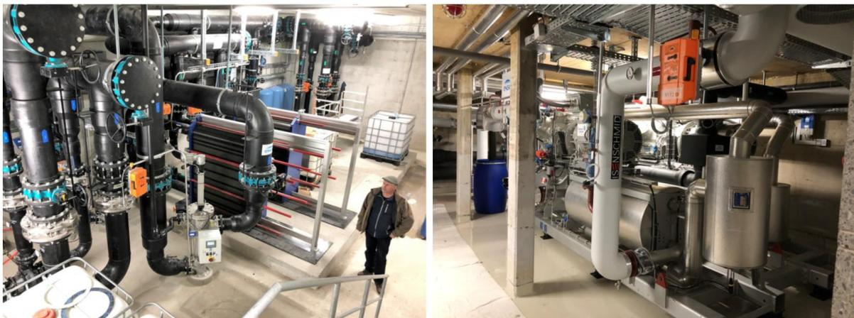
Figure 3. Left: 1 MW Heat pump; Right: Lake water pumping station. (Source: Corporation Weggis).
