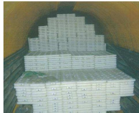
Internal view of the phase change storage tank, the phase change panels are clearly shown
