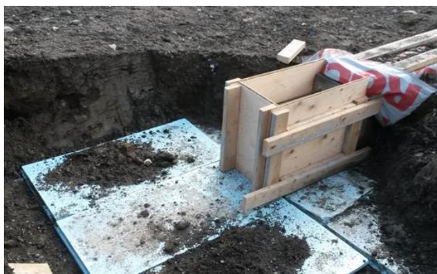
The sketch is from the design stage (courtesy of Bergersen Arkitekter AS), and the photograph (courtesy of Marianne Rose Inman) is from the construction/as-built stage. Note the missing concrete pier foundation and additional insulation.
